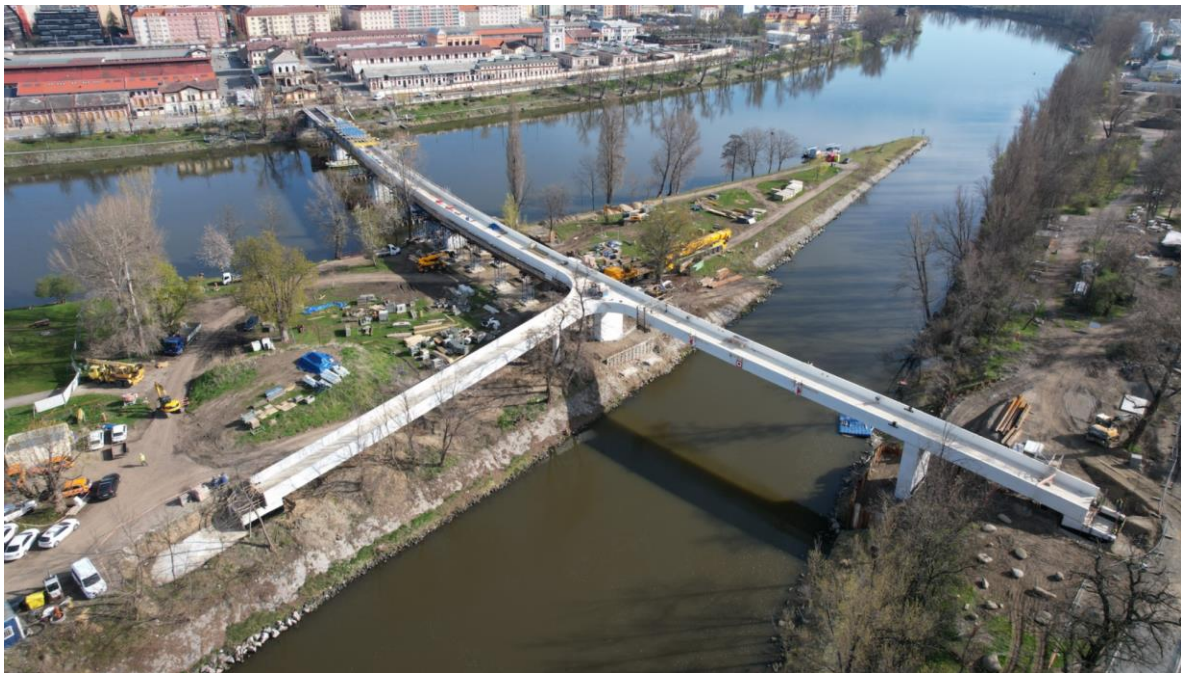
Figure 23. Construction of the footbridge, source: IPR Praha
