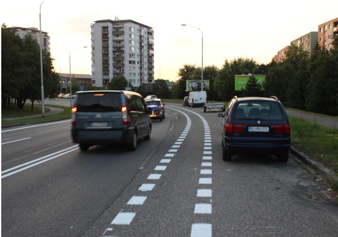
Figure 37: Poorly designed bicycle infrastructure implemented in 2018.
